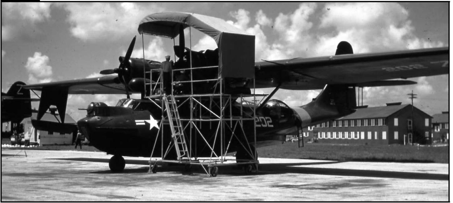
*Here's one for the old timers. Consolidated PBY-6A Catalina (note the taller tail fin in comparison to the shorter PBY-5A tail fin that's just visible at left) "Zulu-Two-Zero-Two" from NAS Squantum's VP-ML-69 is having some maintenance performed on its port engine during an annual training detachment to NAS Miami, FL in the summer of 1950. Many thanks to Joe O'Neill for this photo. Got something similar to share? If so, contact Marc J. Frattasio.*
